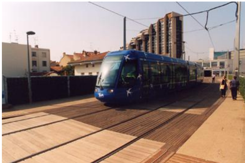
Decking - Tramway track - Montpellier, France (© Michel Vernay)
