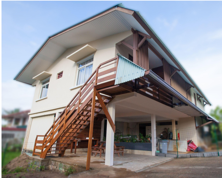
Outdoor staircase in Gaiac de Cayenne, Rémire- Montjoly, French Guiana (© Nicolas Quendez)
