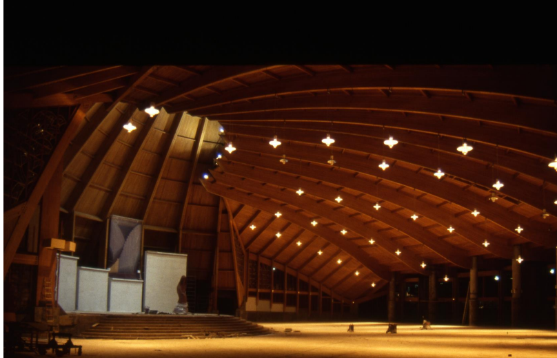
Glued laminated indoor structure at the Mary Queen of the Apostles Basilica in Yaoundé - Cameroon (© Jean Uhalde, UBC).
